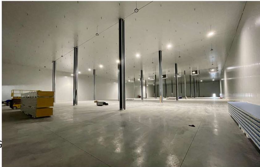
321,000 square feet facility Floor pouring completed earlier in Q3
