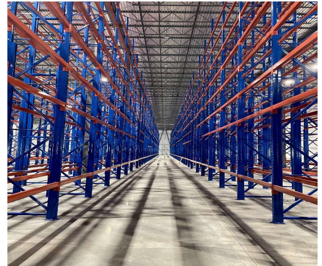
40 feet high ceilings Racking installation in progress
